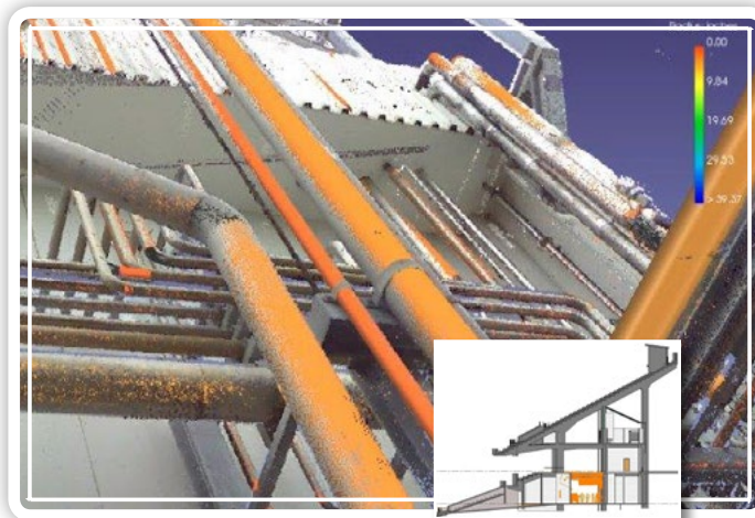
EdgeWise MEP pulled 90-95% of pipes accurately - lengths, elbow angles, and sags in long pipe runs included.
